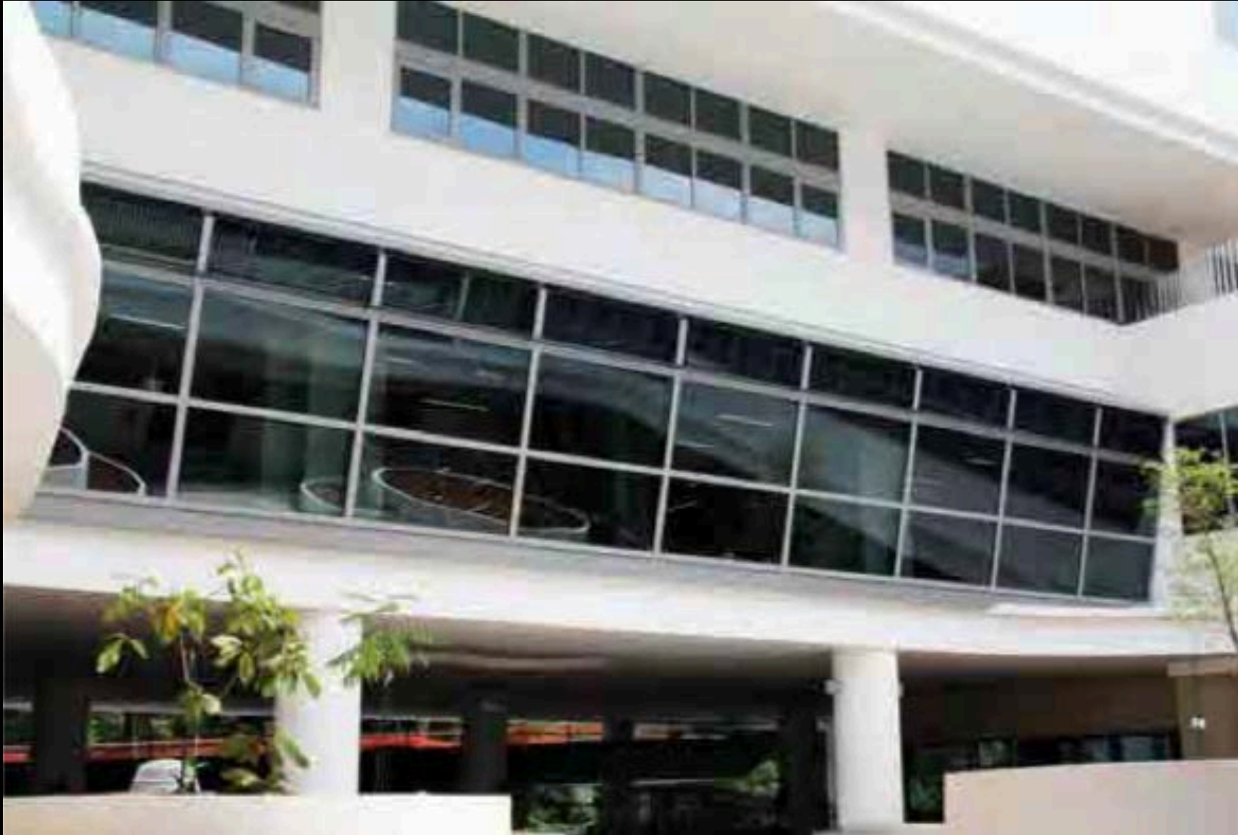
UCWSEA pilot installation, Singapore, 2015
