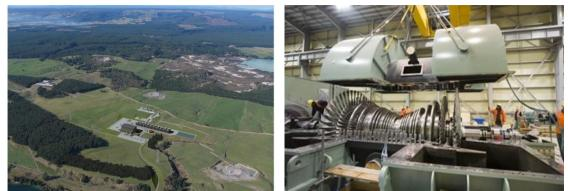
Source of Photograph: Tauhara North No. 2 Trust 2009 Mighty Power River http://202.74.224.54/Generation/PowerStations/Geothermal/NgaAwaPurua/Gallery.aspx Location: Northeast of Taupo Commission Date: 2010 Current Capacity: 140 MW Technical Features: Triple-flash configuration utilizing high, intermediate and low-pressure steam inlets, accommodating the largest single-shaft, custom-made geothermal turbine in the world
