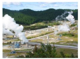
Source of Photograph: Richard Seaman http://www.richardseaman.com/Wallpaper/NewZealand/NorthIsland/WairakeiGeothermalPowerStation.jpg Location: North of Taupo Commission Date: 1958 Current Capacity: 181 MW Technical Features: Wet steam plant (the original main plant). Binary plant addition in 2005 to utilize low temperature steam from the main plant
