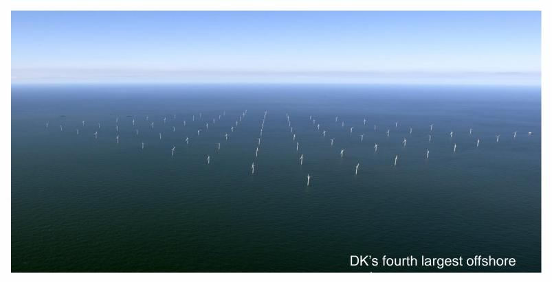
$80 \times 2$  MW turbines at water depths 5-15 meters. Production 600 GWh/year equals the electricity consumption of 150.000 households.
