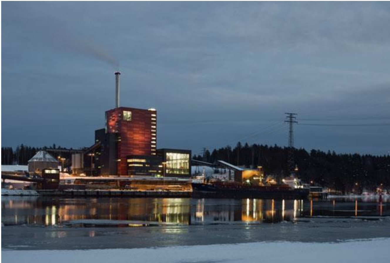
Igelsta plant in Södertälje, 200 MW heat, 75 MW electricity (source: Söderenergi)
