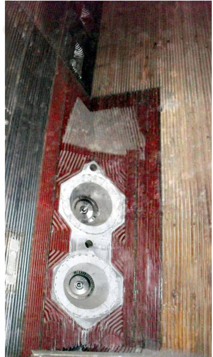
Burner configuration In the corners
