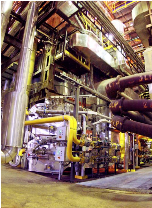
Water tube boiler CHP, tangential fired
