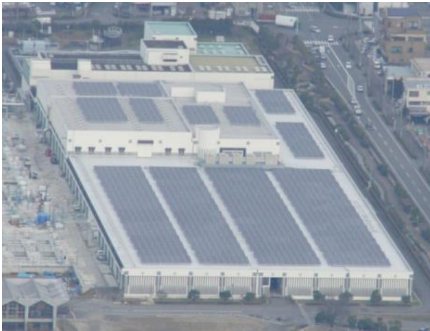
Toba Treatment Plant
